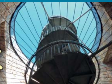
Spiral staircase in the Hausmannsturm
