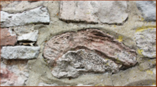
Roe-limestone and a stromatolitic buildup (centre) as building stones in the Rid-dagshausen monastery
