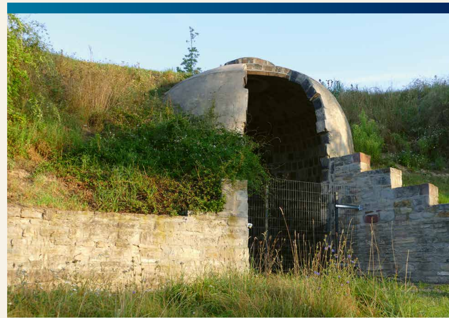
Secured remains of an underground grain silo with a subsequently erected reinforcing wall
