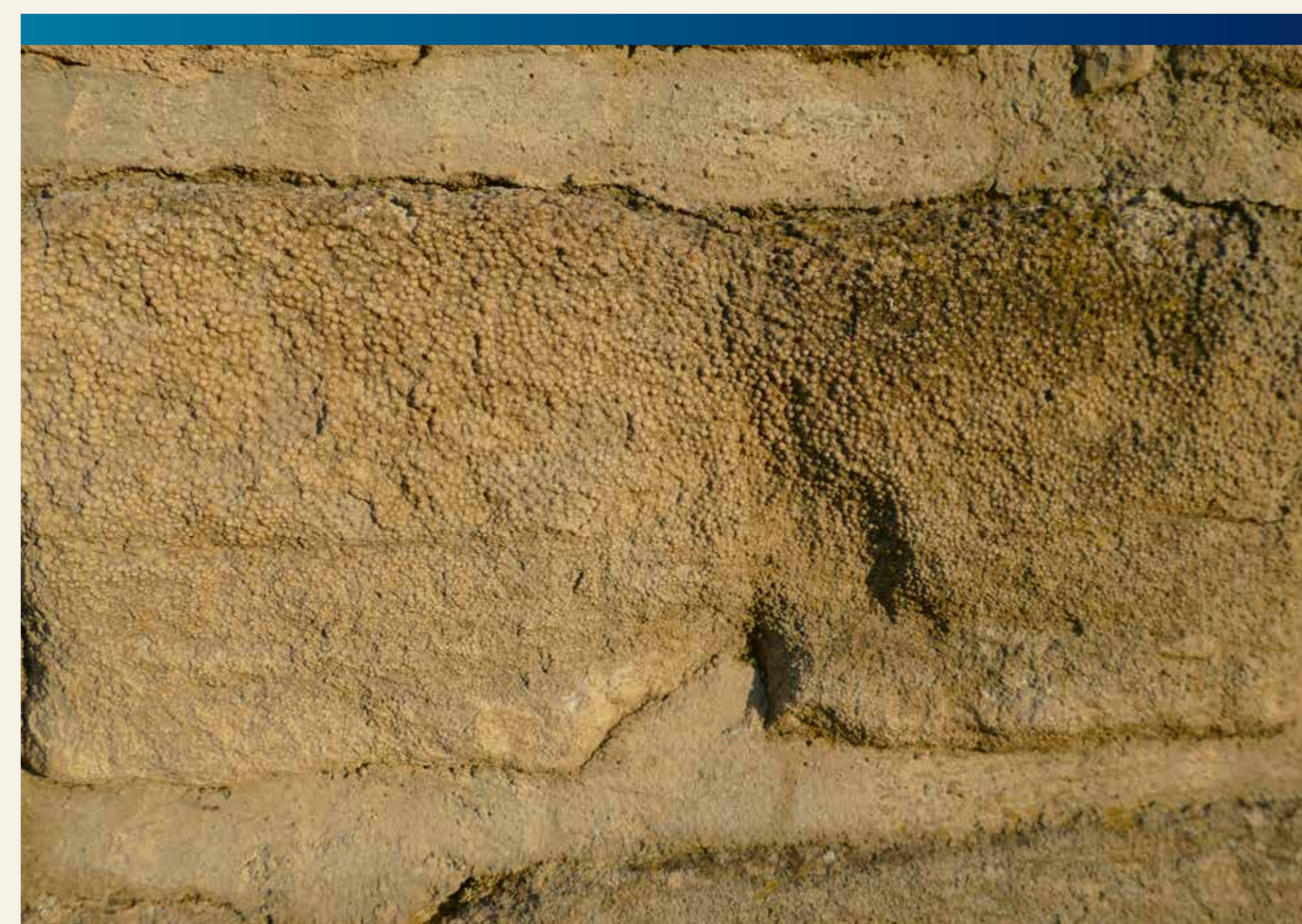
Oolitic limestone from the Mansfeld basin: the primary building material in the reinforcing wall
