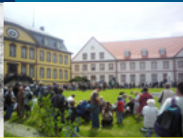
Remaining buildings of the Dorstadt
