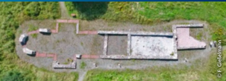
Aerial view of the foundations of the chapel with intermediate building and floor screed
